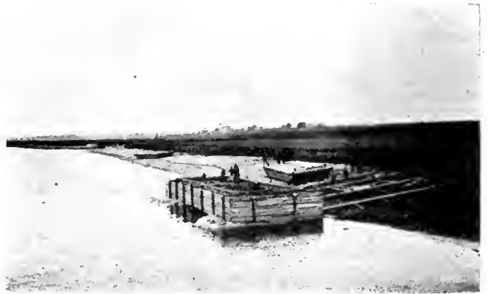
Fig. 4.—Launching caisson for pier No. 3.
